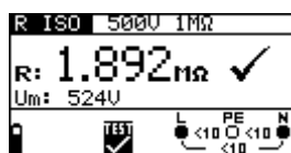
Figure 5.3: Example of insulation resistance measurement results
